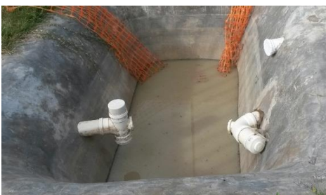
After -Water pit-
